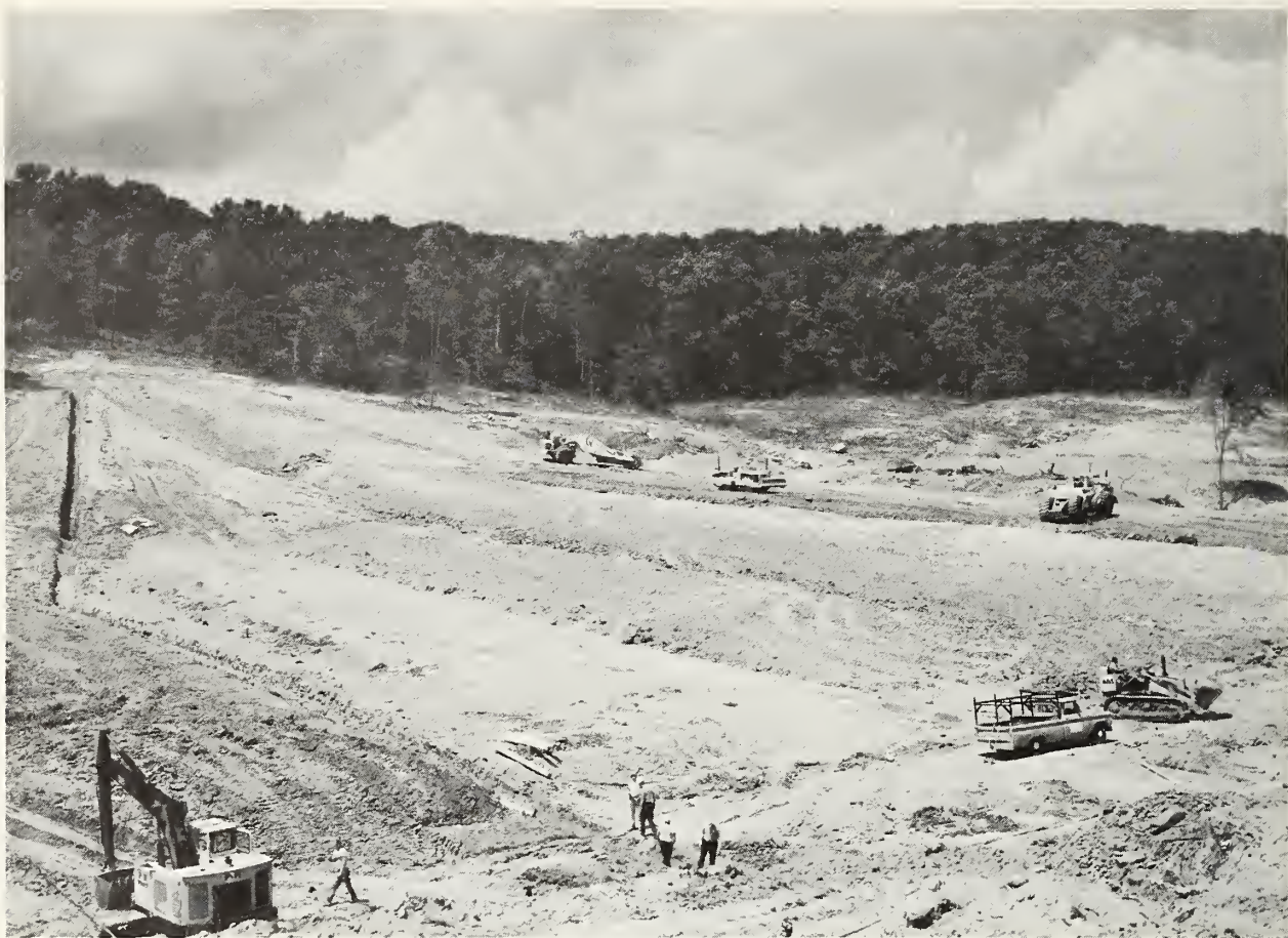
The initial benefits will be realized from construction.
